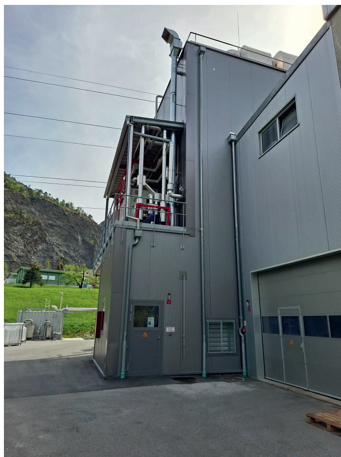
Fig. 6. Exterior view of the phosgene bunker at the Valsynthese production facility.
